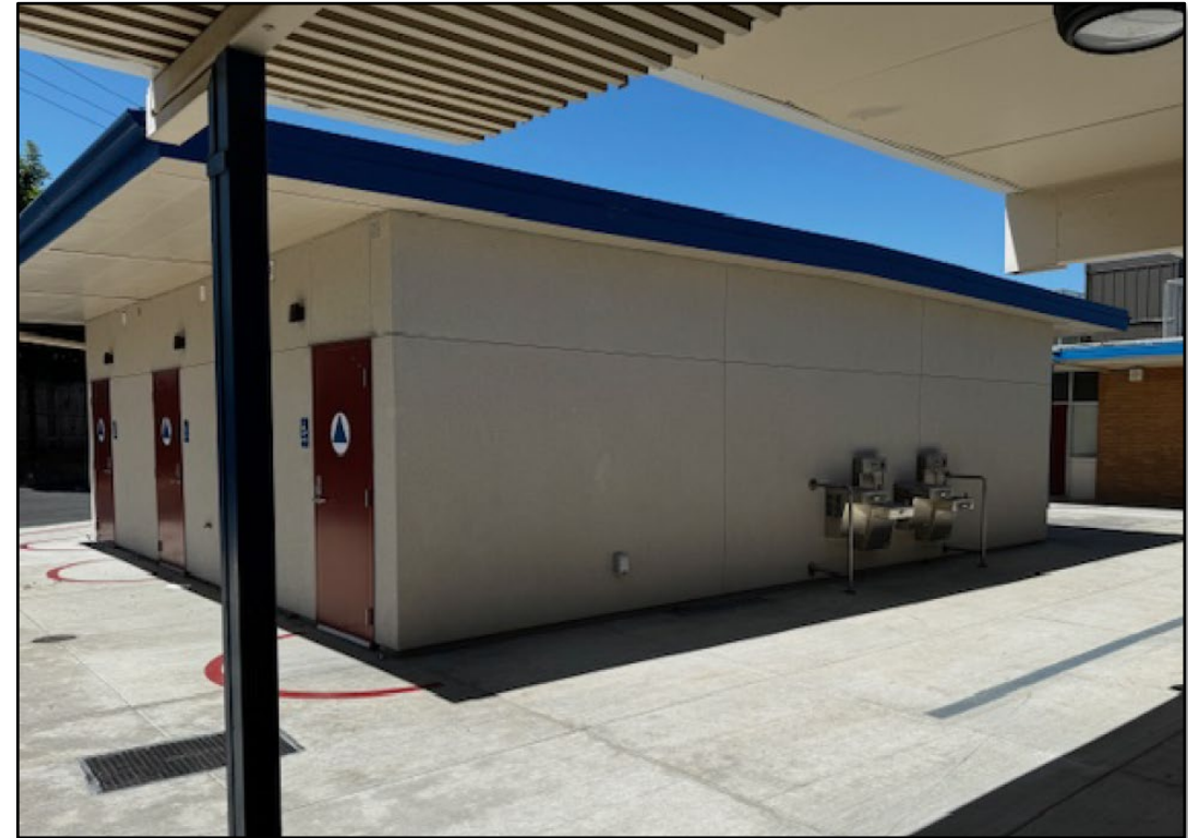
Frontier ES Restroom (New)
