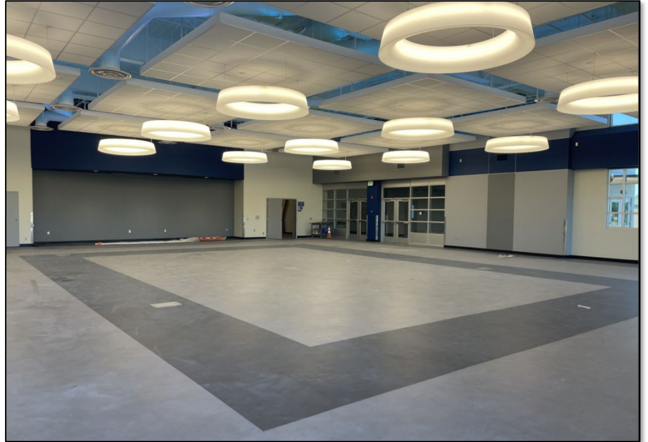
Norwood JHS Cafeteria (Progress)
