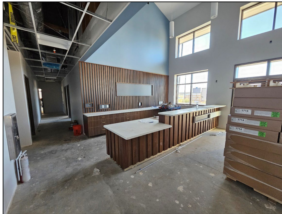
Northlake TK-8 Admin Office (Progress)
