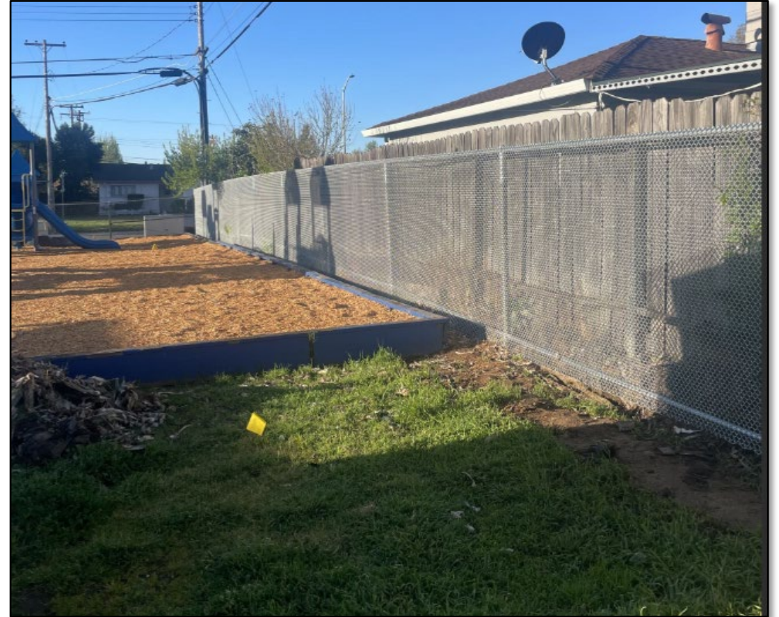
Fairbanks ES Fencing (Progress)
