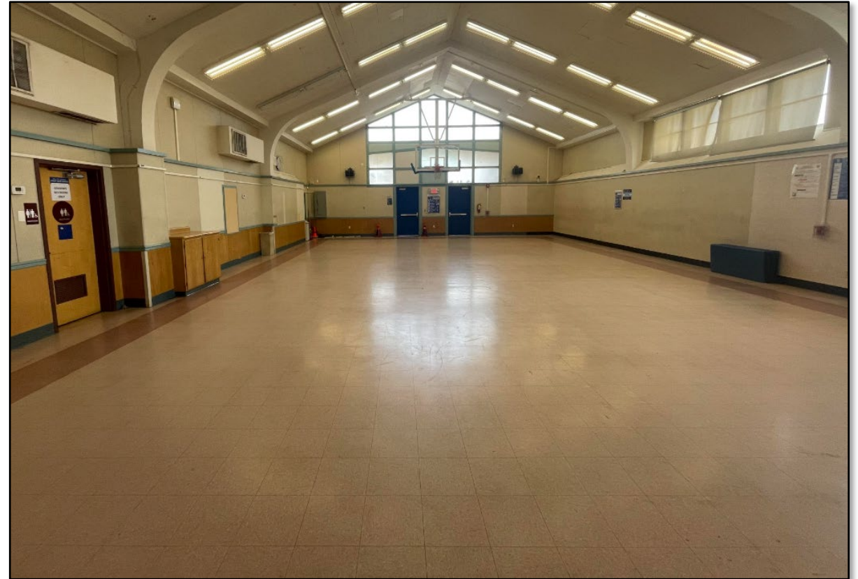
Oakdale ES MP Room Flooring (Existing)
